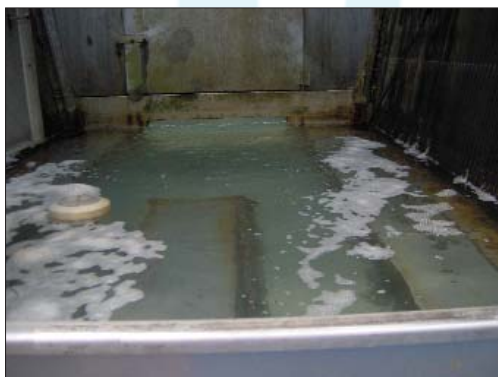
Cooling Tower Sump
